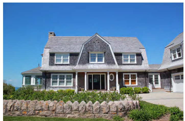
Example of modern construction on Chapoquoit Island which incorporates elements of Shingle style such as a cross gambrel roof and wood shingles
