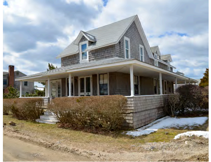
Example of camp-meeting house with shingle siding and wrap-around porch in Menauhant
