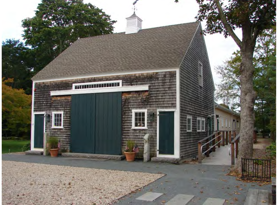
Adaptively reused stable at the Falmouth Historical Society
