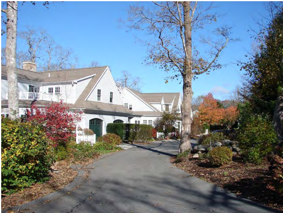
Condominium project sensitively set into a woodland in West Falmouth and screened from the adjacent public road
