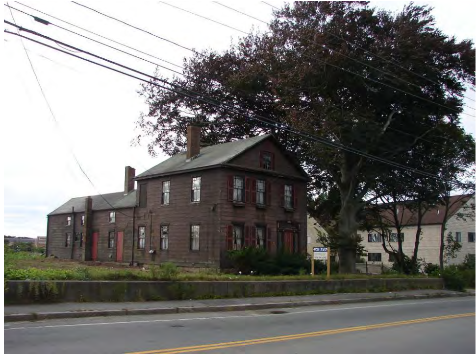
Threatened building on land to be developed along Route 28
