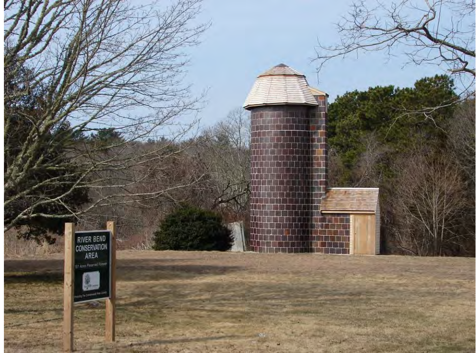
Preserved silo at River Bend Conservation Area
