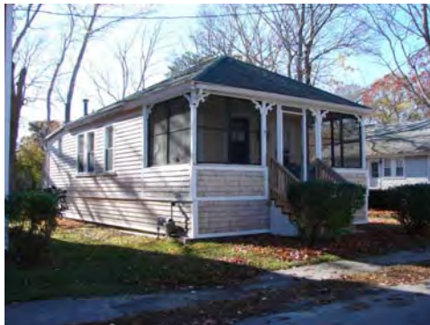
Cottage in a residential neighborhood
